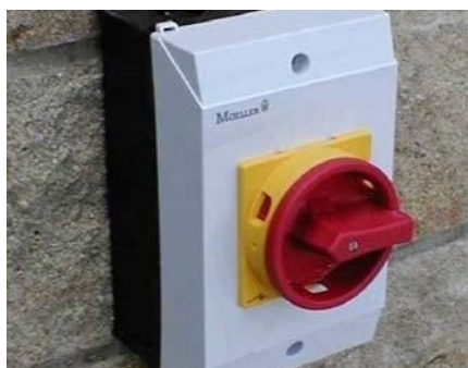
Rotary Isolation Switch
