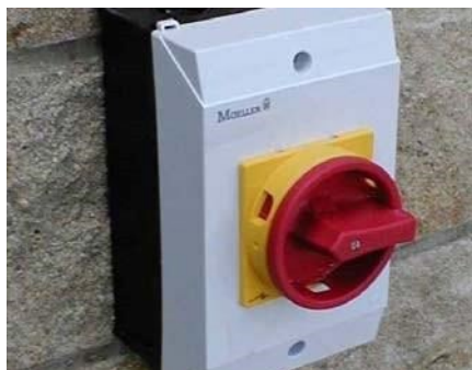
Rotary Isolation Switch
